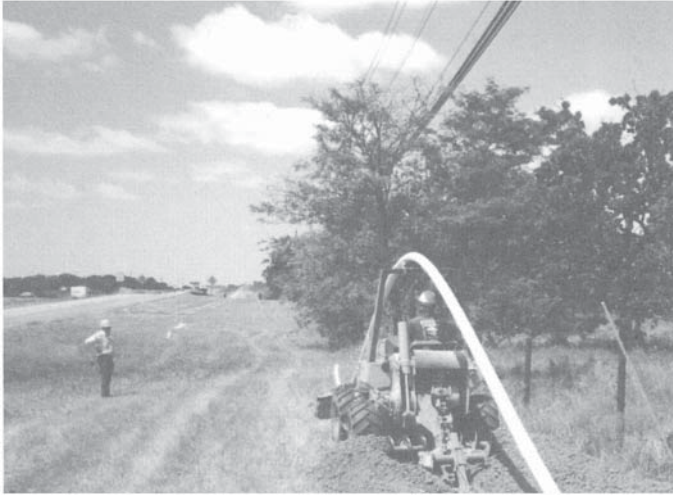
Fig. 2. A cable plow places optical fiber duct in a single operation.
